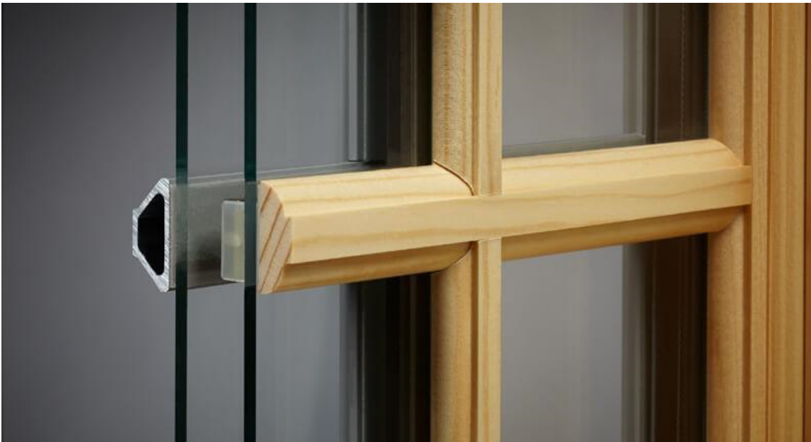
Figure 5.3 - Image of Simulated Divided Lite (SDL) window. Both inside (shown in wood) and outside (shown in hollow metal) muntin's are applied to double pane glazing (glass).
